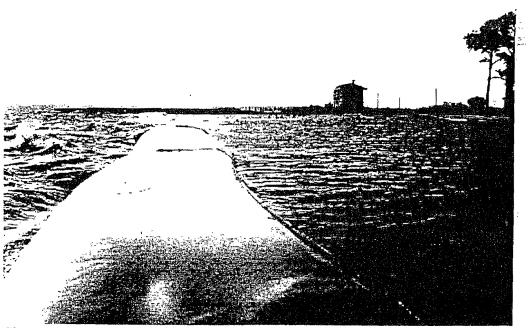
Figure 4. Variation in the alignment of a geotextile tube
